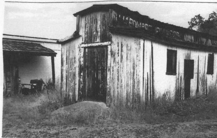
Maxville House behind Oddball Junction
